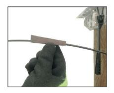
Place the flat cable on the bootom of the clamp body.
