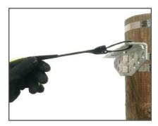
Hang the bail wedge onto the hardware fitting, lock the bail.
