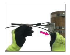
Position the shim onto the cable in the clamp body, with the gripping bumps facing the cable.
