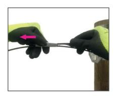
Pass the wedge in the large section of the clamp body then initiate the clamping onto the shim + cable.
